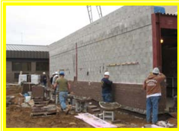
Exterior masonry in progress at auditorium addition
