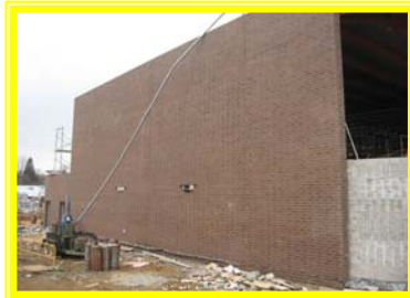
Exterior masonry in progress at auditorium addition
