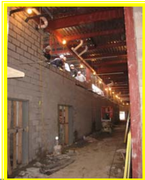
Corridor wall masonry in auditorium addition
