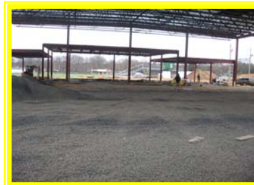
Slab pours and preparation work Gym Addition
