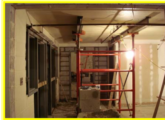
Music area renovations underway
