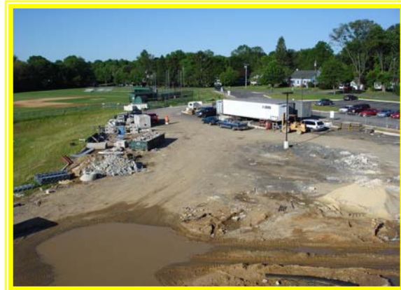
Parking lot clean up
