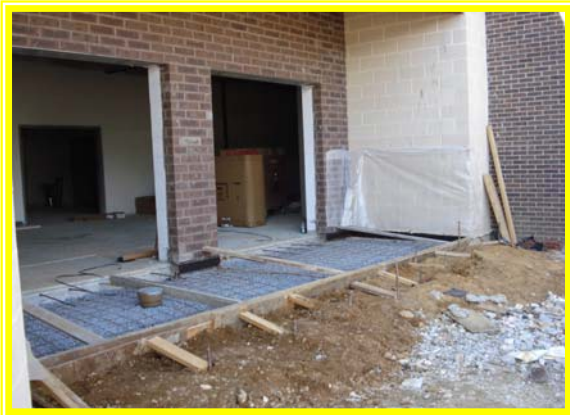
Concrete pads at doorways
