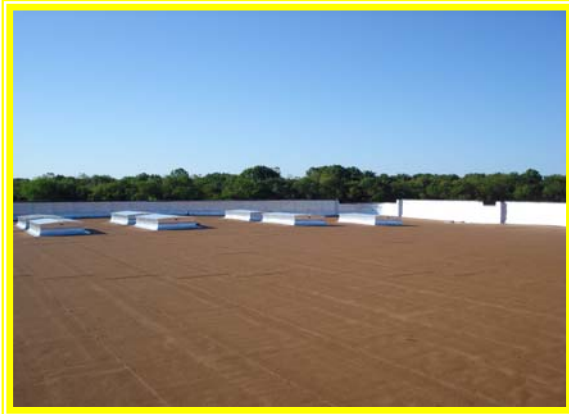
Auditorium roof nearing completion
