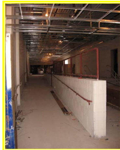
Gallery corridor in progress
