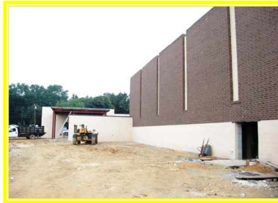
Site work progress
