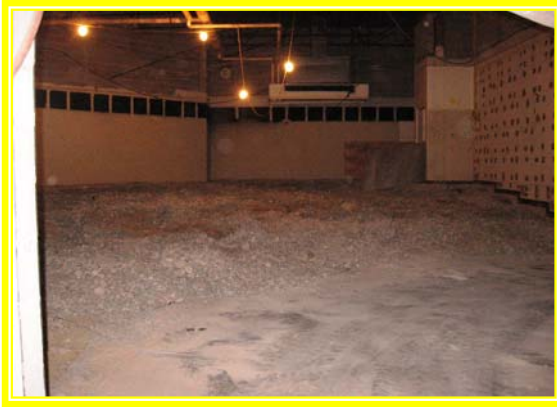
Art Area renovations underway- removal of existing tiered music floors
