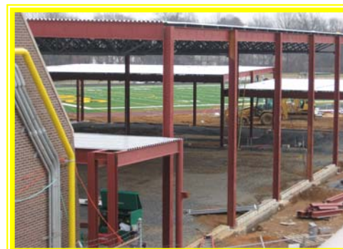
Steel erection completed at Physical Education addition
