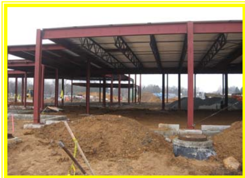
Steel erection completed at Physical Education addition
