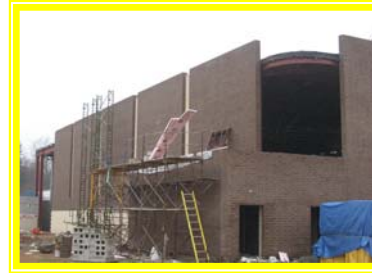
Auditorium addition progress
