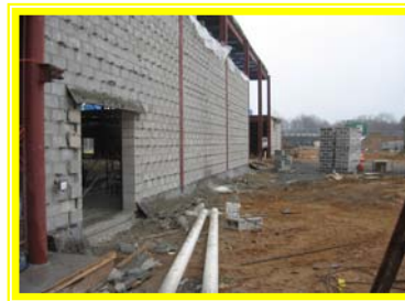
Gym addition progress
